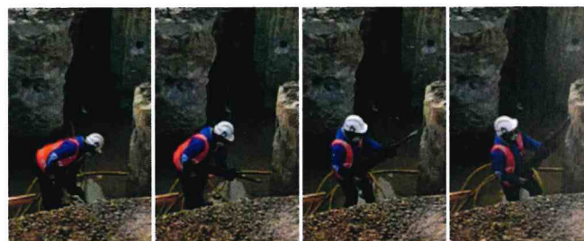
FIGURE 2: Lifting the jackhammer into position* REFERENCE(S): 7.2.2, p. 175.
