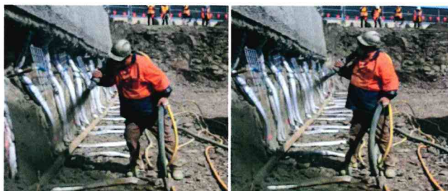
FIGURE 5: Manual shotcreting* REFERENCE(S): 5.3.2, p. 131.
