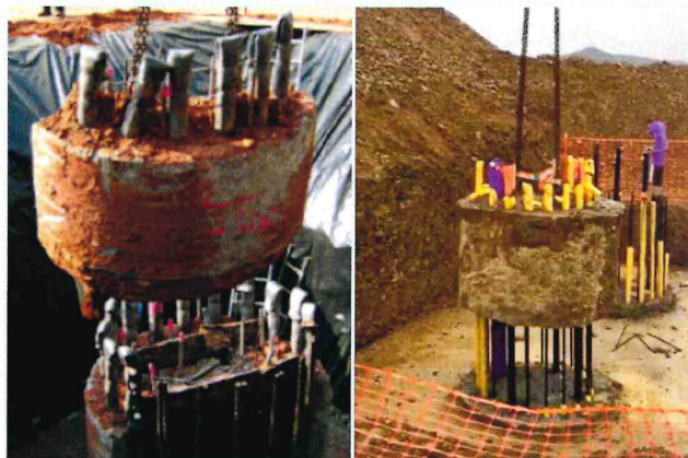
FIGURE 4: Alternative chemical pile breaking method 2
